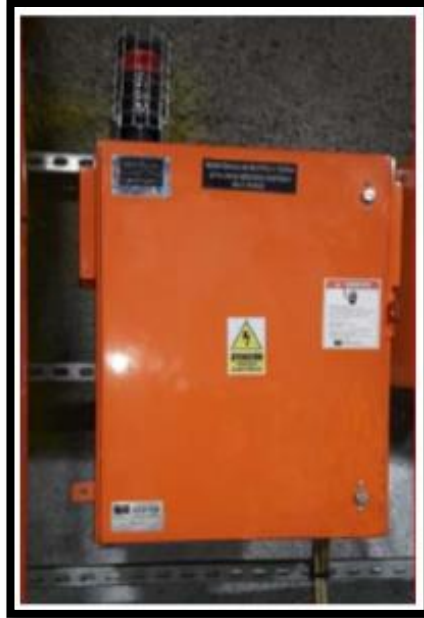
Figura 22. Tablero porta Ground Check
