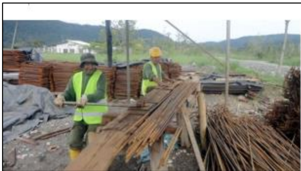
Figure 1. Manual bending of rods
