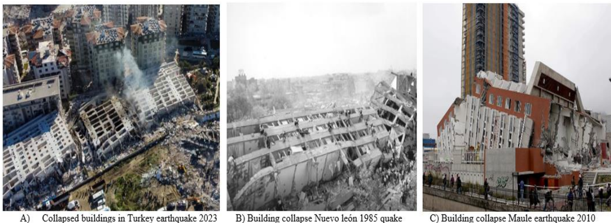
Figure 1. Collapse of buildings in different countries due to seismic events
