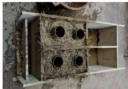
Fig. 8. Assembly of the lightened block.
