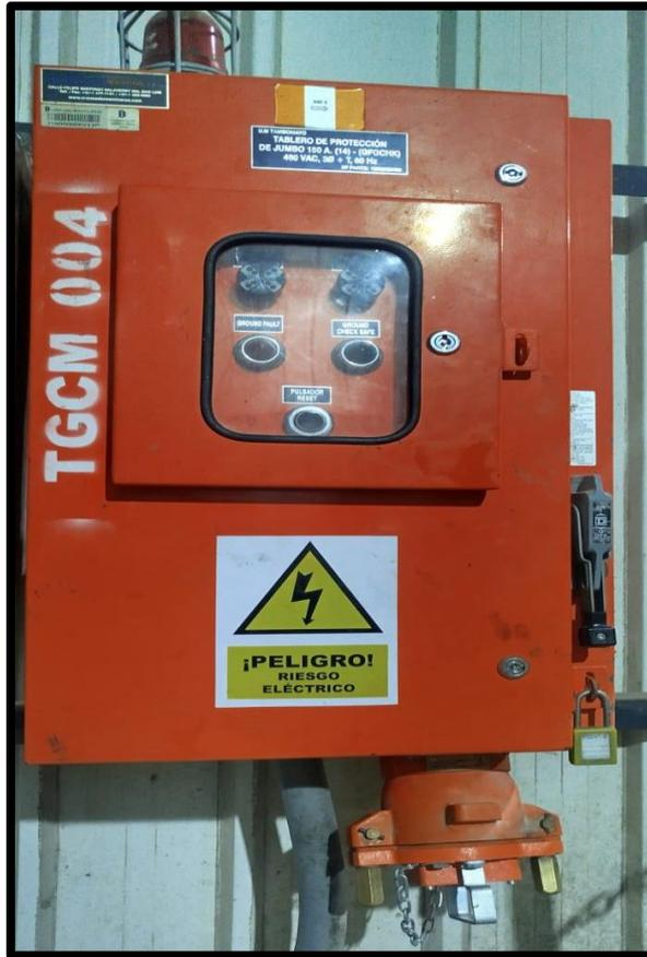
Figura 21. *Tablero Ground Fault y Ground Check.*
