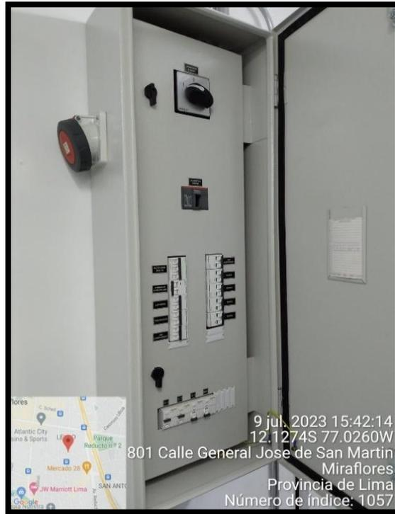
**Figura 27. Tablero general instalado**
