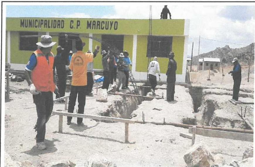
FOTO 08: ZAPATAS, CONCRETO FC=175 KG/CM2
