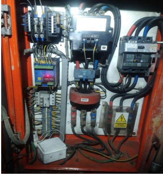
Fig. 10 An AIoT system installed in a 50 HP underground pumping chamber
