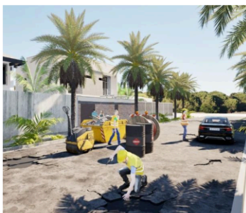
Figure 11. Repair of rigid pavement
