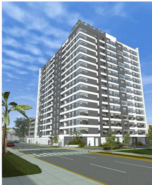
Figura 6: Edificio Atlantik Ocean Tower, San Miguel – Lima
